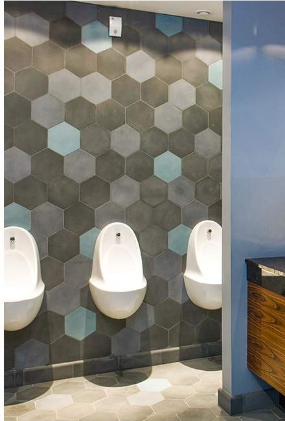
Hotel restaurant and bathroom area tiled with 20x23cm hexagonal tiles in a combination of 3 cement colours (GL, GPL & G2)
