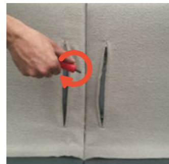
Completely tighten nuts in both backs. Apretar los 4 de los respaldos.
